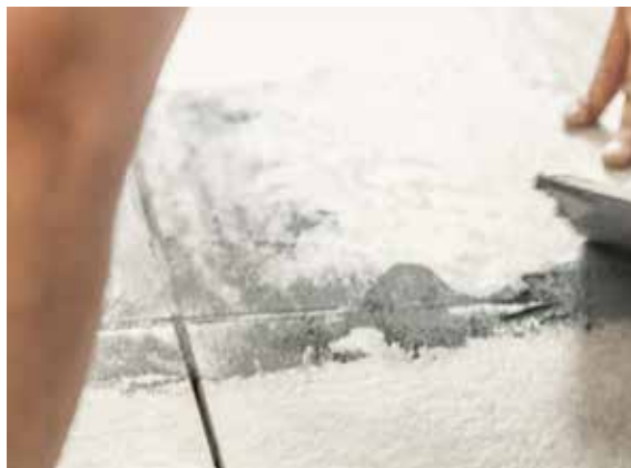
4 Grout the tiles using special system grout mortar. Ensure the correct mixing ratio of grout mortar and water as per manufacturer's instructions.
