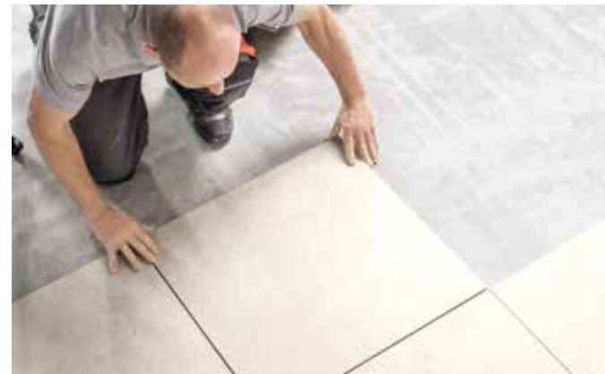
3 Specify the joint grid and lay the cork edges tightly against each other.
