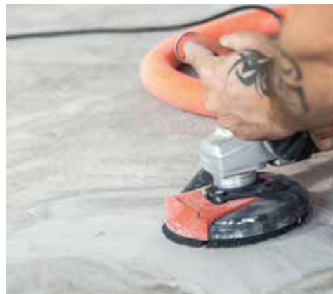
2 Rework the floor if necessary in order to ensure the requirements on evenness.
