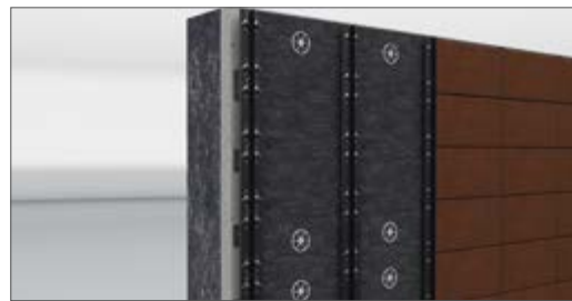
Mount the T-profile with approved fastening means
