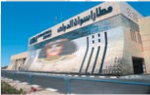
■ Airport, Assuan, Egypt
