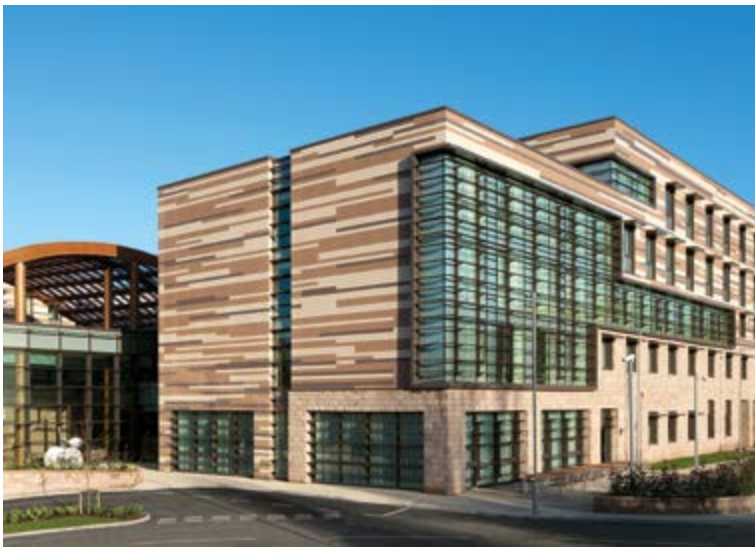
Orchard Hotel, Nottingham, Great Britain / Architect: RHWL Architects / Photo: Martine Hamilton Knight Photography / BREEAM EXCELLENT
