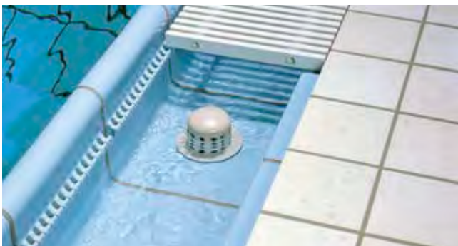
Flüsterrinne Wiesbaden Silent Wiesbaden Silent low-noise channel
